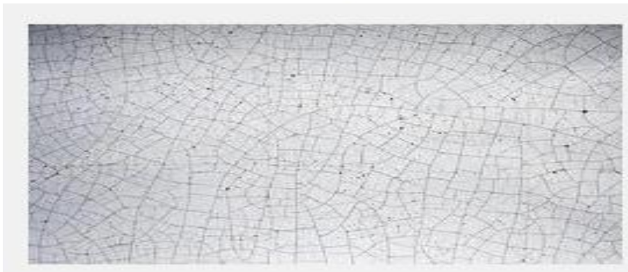
Cracks in plaster
